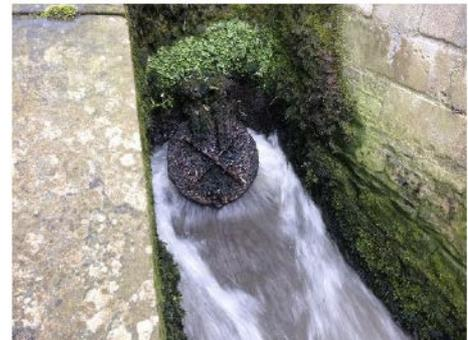
Figure 2: Treated effluent outfall
